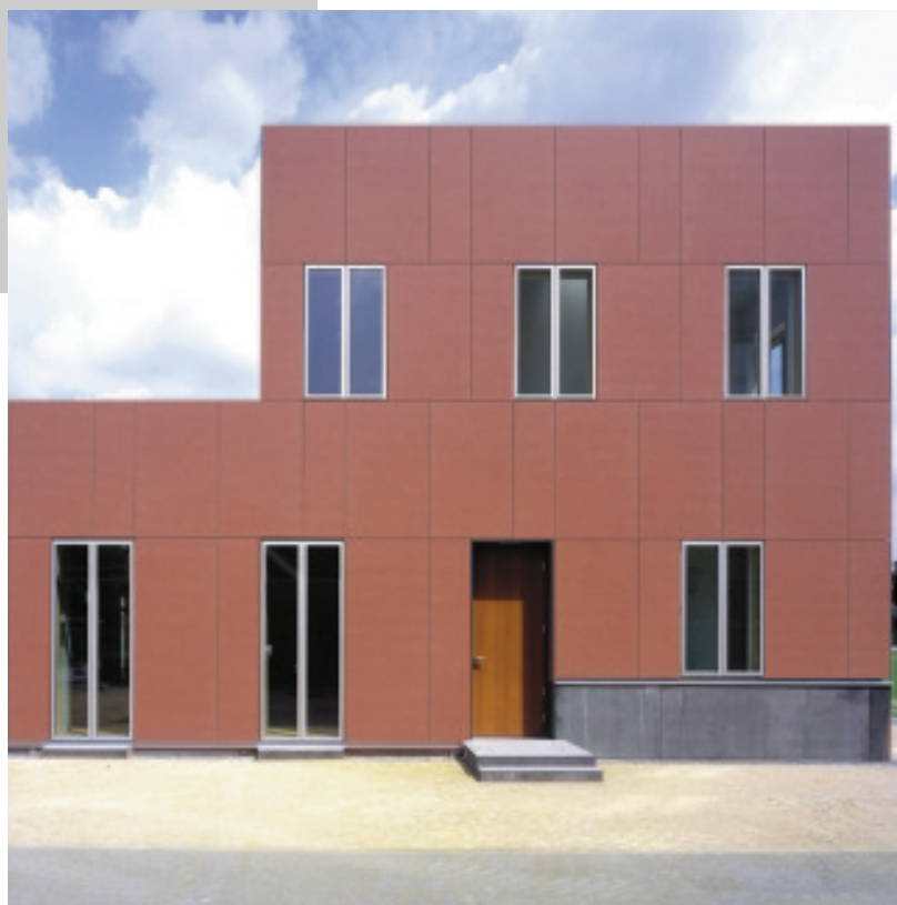
CLADDING WITH FIBRE CEMENT
